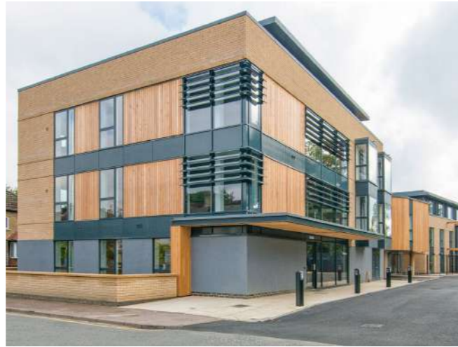
4- LUCY COLLEGE STUDENT ACCOMMODATION - 4 STOREY
