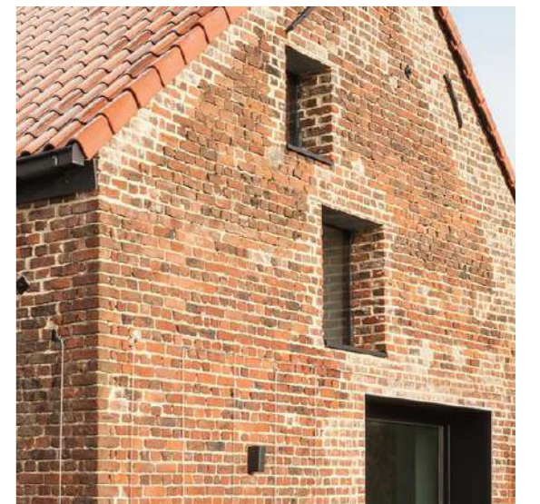
IRREGULARLY ARRANGED FENESTRATIONS
