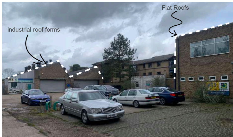
EXISTING BUILD FORMS
